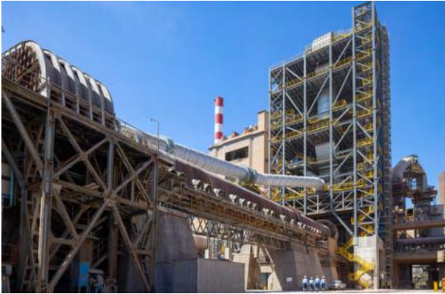
Precalciner unit at Kamari cement plant, Greece.
