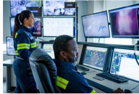
Control room at Pennsulo cement plant, USA.
